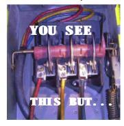
Often, a common cause of such insidious faults can be due to hidden corrosion between the mating surfaces of electrical terminations. Other causes may include; Loose terminations caused by bad installation, vibration, and/or inductive and thermal changes, Faulty manufacture, Burnt contacts, Insulation break down, Occasional overloading, Neutral Harmonics, Partial cooling system failure, Weather exposure, etc.
