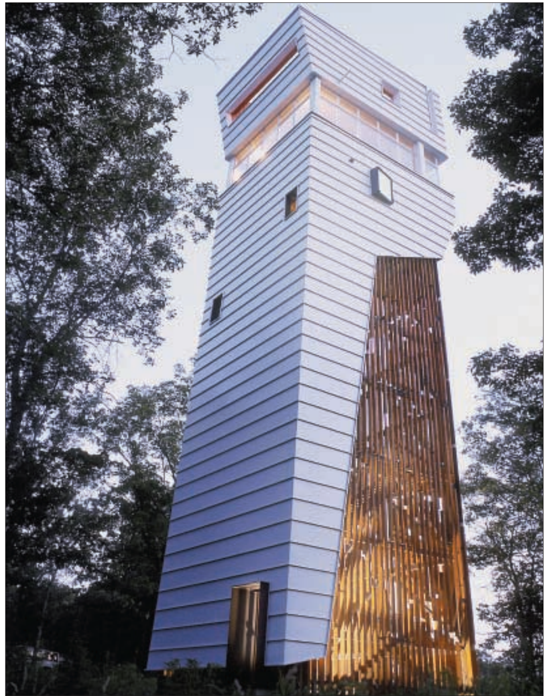
PHOTO COURTESY OF THE UNIVERSITY OF ARKANSAS The Keenan TowerHouse, an 80-foot-tall structure similar to a fire tower, stands above the tree canopy near Old Wire Road in Fayetteville. The tower, which has been the subject of recent television shows and magazine articles, was built using white oak, river stones, pecan shells and locally fabricated steel.
