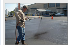
Coal-tar-based sealcoat being applied to a test plot.
