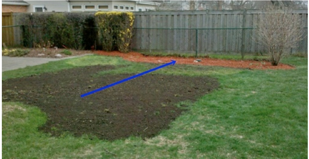
Figure 16: Grading water into the rain garden.
