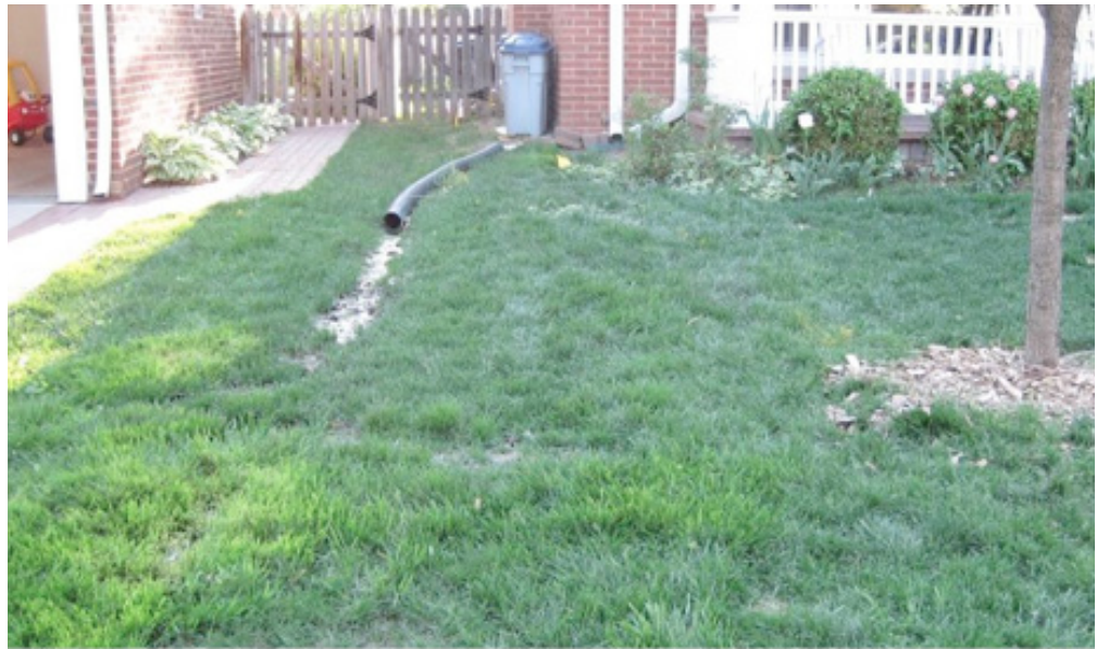
Figure 8: Sump pump outlet causing standing water issues.
