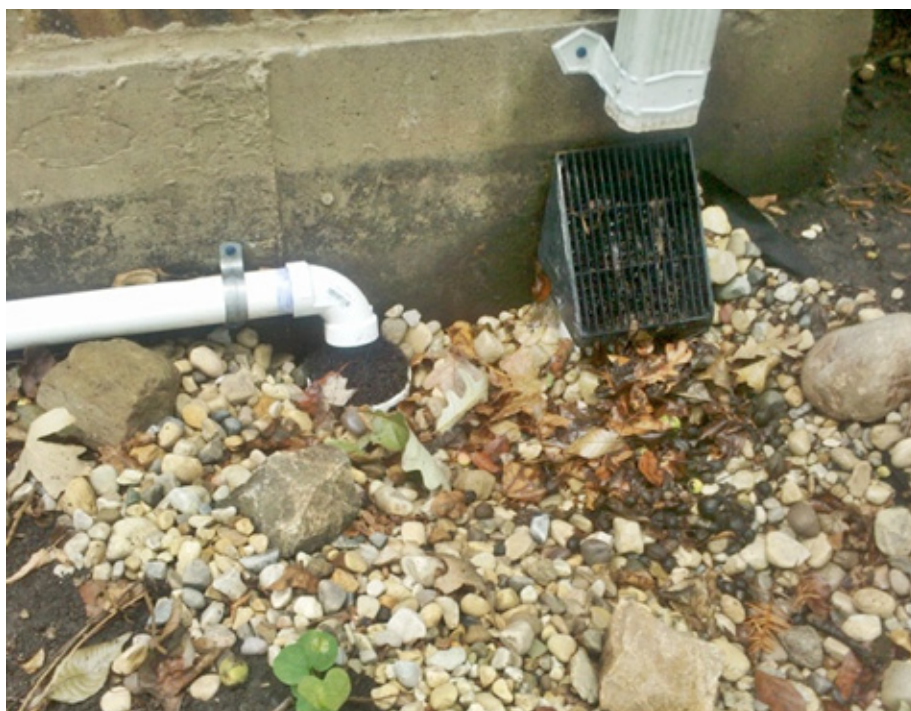
Figure 17: Sump pump line to the left directed into PVC pipe with foam filter. Downspout in the upper right that is directed into leaf filter.
