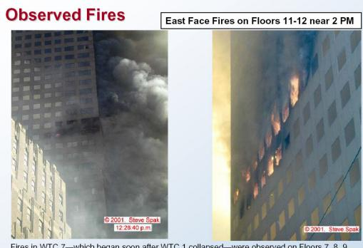
Fires in WTC 7—which began soon after WTC 1 collapsed—were observed on Floors 7, 8, 9, and 11 near the middle about half an hour before collapse; Floor 12 was burned out by this time. Fires were also seen on Floors 12, 13, 22, 29, and 30 at various times during the day.
