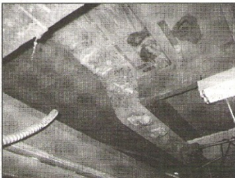
Masonry wall removed
