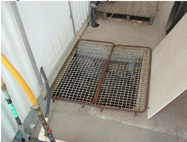
Floodwater that collects and saturates the ground finds its way into the crawl space and takes many days to disappear.
