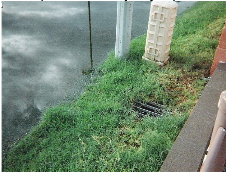
As seen in this photo the floodwater is unable to drain since the drain inlet is well above the level the water.
