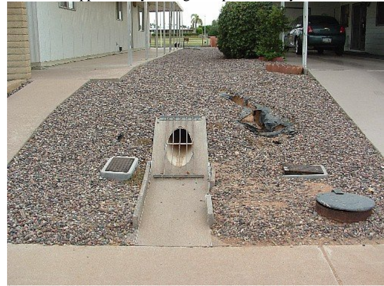
The drain outlet empties onto N. Higley Road, but does not serve its purpose since the floodwaters never reaches the drain inlet.
