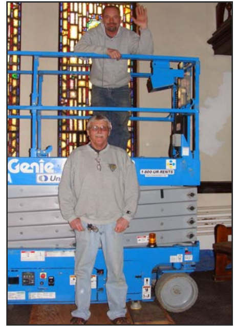
Tim O'Brien and Phil Cereceres Plaster repair in the Hallamor
