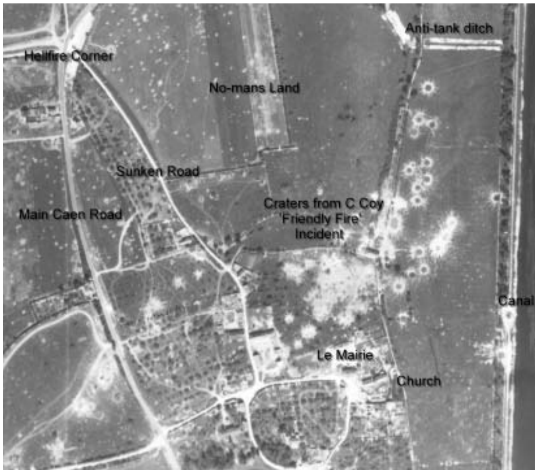
Aerial photograph showing the bomb craters from the friendly fire incident
