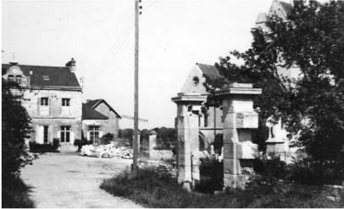
Photo of the square taken looking North with the church on the right and the Mairie straight ahead (notice the rubble). Autumn 1948.
