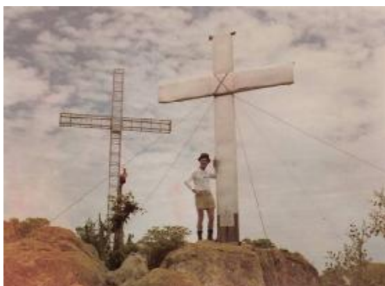
Mt Inungu: The old cross erected by Fr Renk in 1964, with the new cross under construction in the background.
