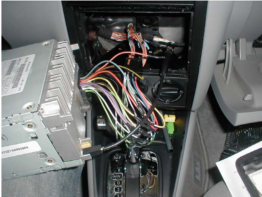
All wires and cables connected
