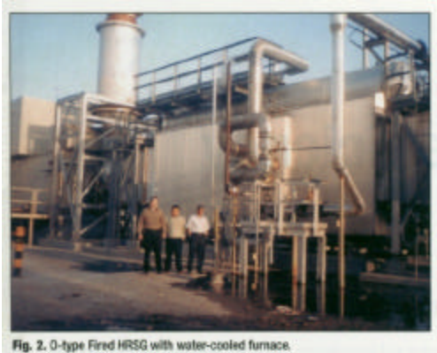
Fig. 2. 0-type Fired HRSG with water-cooled furnace.
