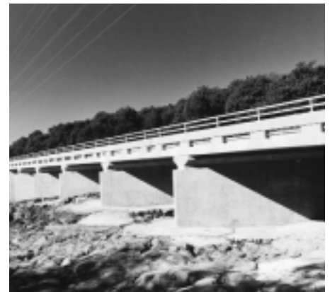
Keaiwa Stream Bridge Replacement Project.
