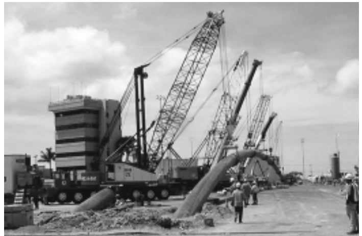
Hart Street Wastewater Pump Station Force Main Replacement Project.
