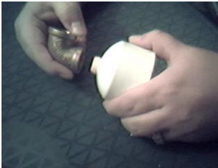
Fig. B Install Elbow
