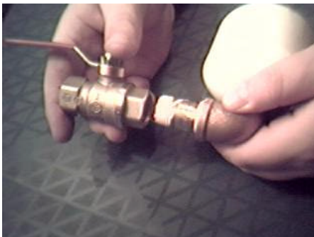
Fig. E Install Valve
