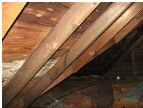
5.0 ROOF FRAMING Picture 1
