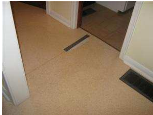
8.2 FLOORS (FRAMED) Picture 1
