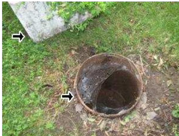
3.3 SITE GRADING Picture 1
