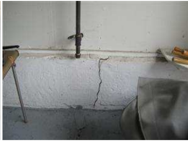
4.2 FLOOR SLAB Picture 2
