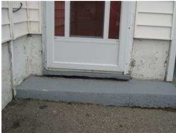
2.2 ENTRY DOORS Picture 1
