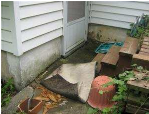
2.3 STAIRS / STOOPS Picture 1
