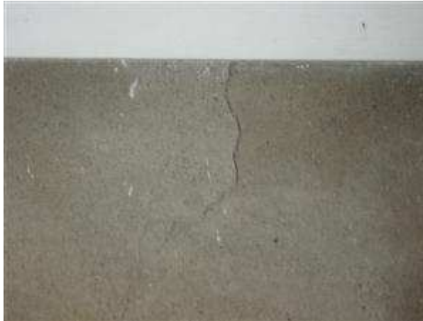
2.6 FOUNDATION SURFACE Picture 1
