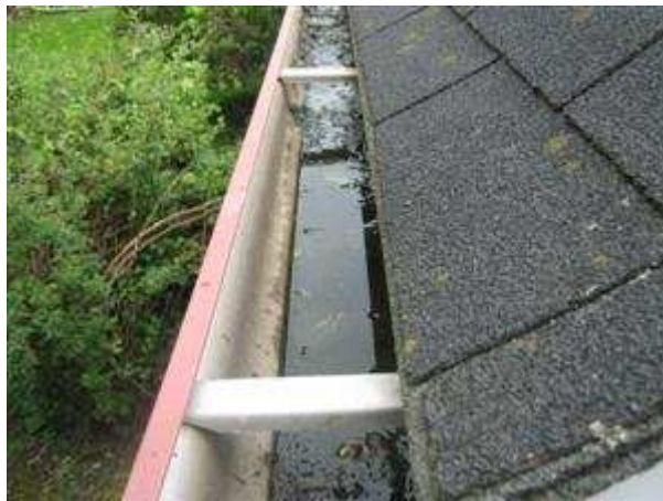
1.5 RAIN GUTTERS / EAVESTROUGHS Picture 1
