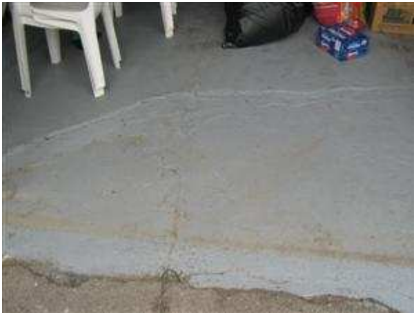
4.2 FLOOR SLAB Picture 1
