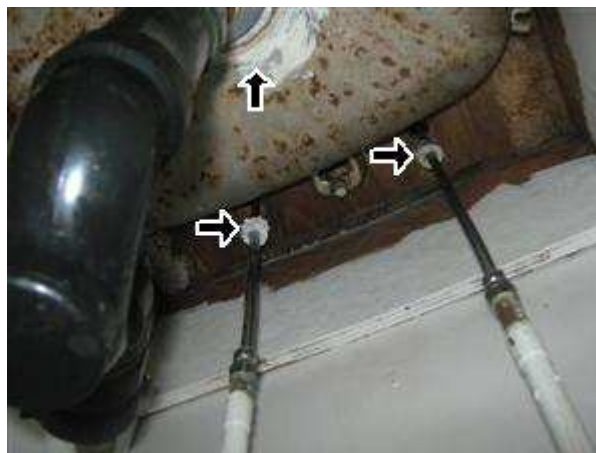
7.0 PLUMBING / SINK Picture 1
