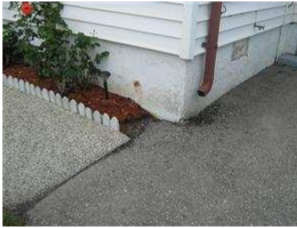
1.6 DOWNSPOUTS / ROOF DRAINS Picture 1
