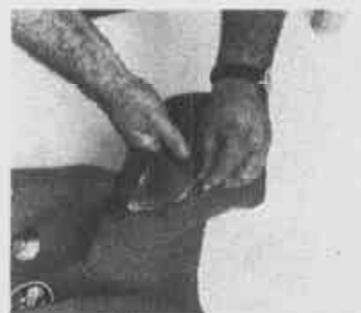
34. Pinch opposite sides of the seam together strongly to ensure a tight bond.
